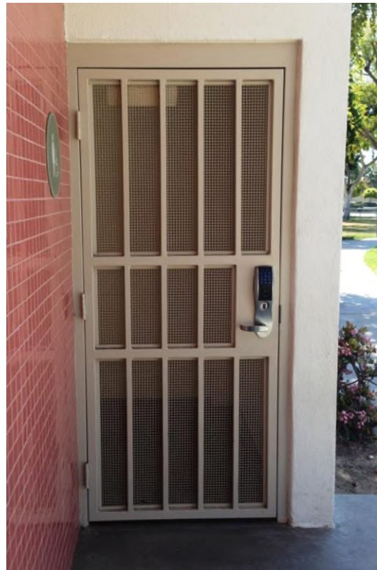
Gate Cross Bracing
