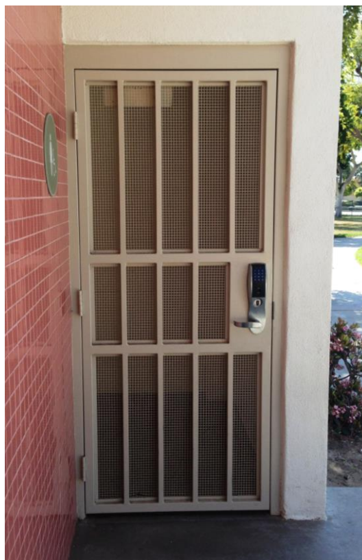
Gate Cross Bracing
